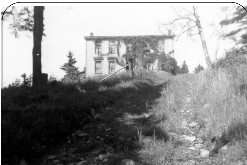
Farrant Home—taken from Farrant Road with the Hugonin-Perrin Carriage Road to right
